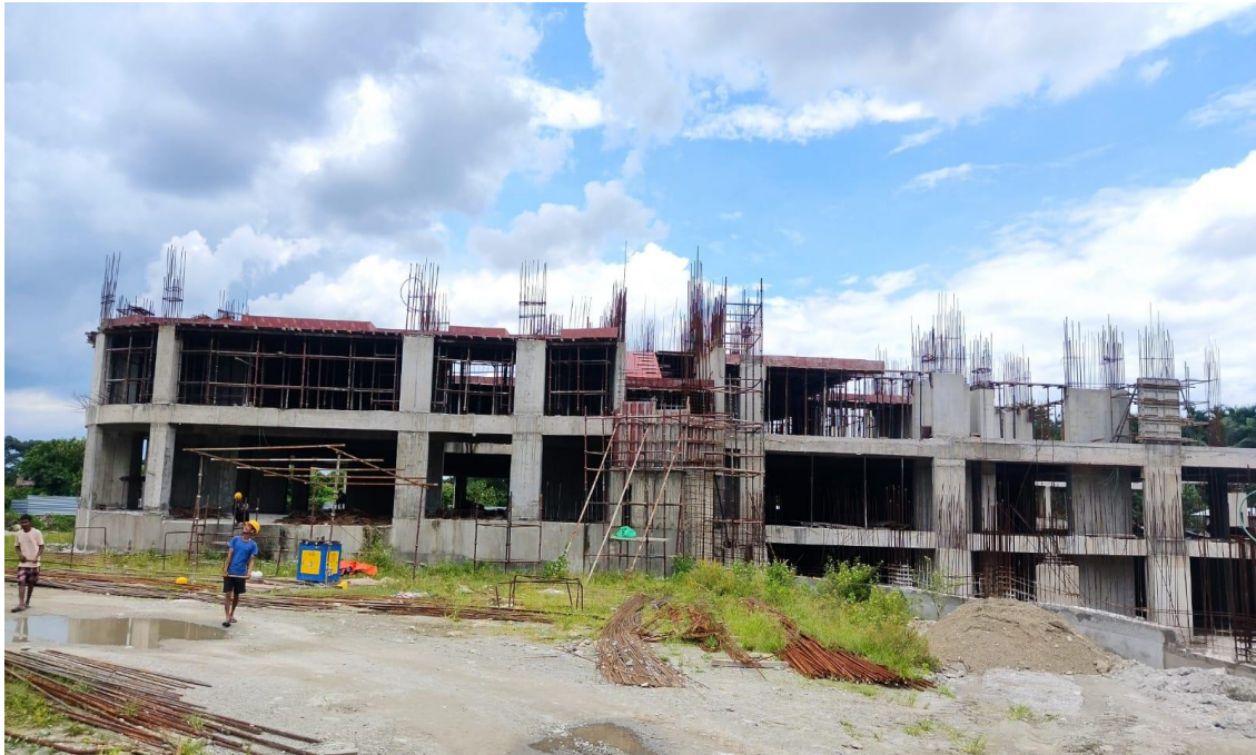
Note: Slab suttering (WIP).
